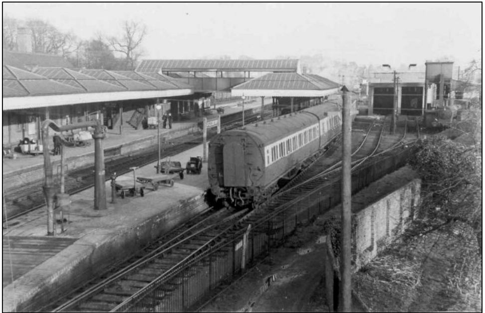
A view of Aylesbury Town station looking in the up direction. This side of the island platform was used by the Princes Risborough service. The loco shed is on the right. photo : GCRS Collection
