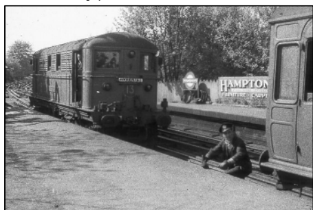
A quick loco change at Rickmansworth. Electric no.13 has brought the train from Baker St and is being replaced by steam for the last stage of the journey to Aylesbury. Dewi Williams Collection
