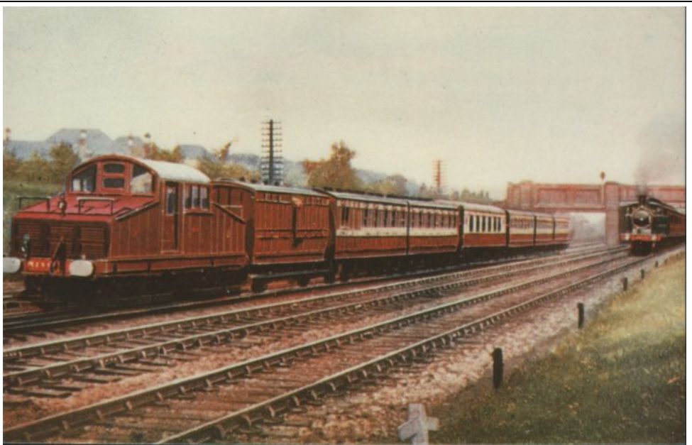
The colour postcard referred to by David Wrottesley on p.34 in Forward 149. It shows a Met Rly British Westinghouse electric locomotive of 1905 hauling a six car train along the Met/GC Joint route to Aylesbury. A Pullman car is included after the 2 nd coach. On the right a GC train also heads north on the non-electrified tracks.
