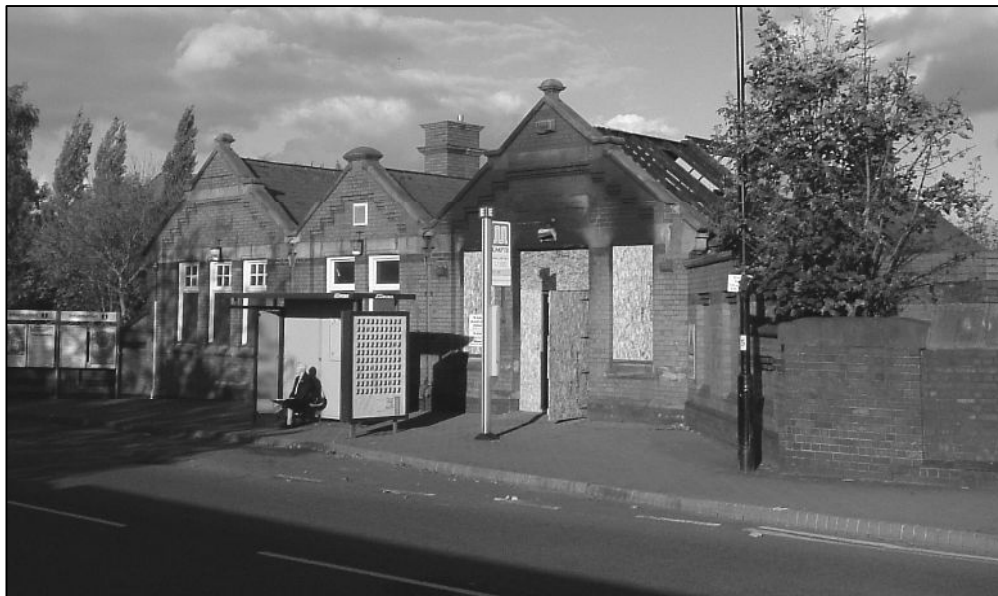
Guide Bridge station after the fire of 19 October.
